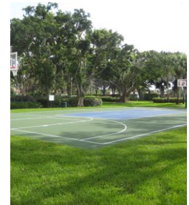
New Basketball Court
